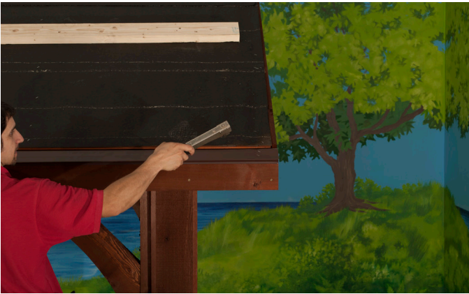
Fasten with Hammer Stapler or 1" Shingle Nails every 2 feet.
