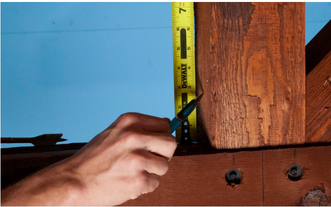
Using the previous measurement, mark the center of the Vertical Web.
