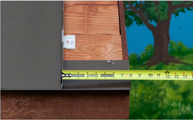
Measure distance from edge of Metal to edge of Roof.
