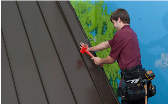
Using previous steps cut and bend the last Piece.
