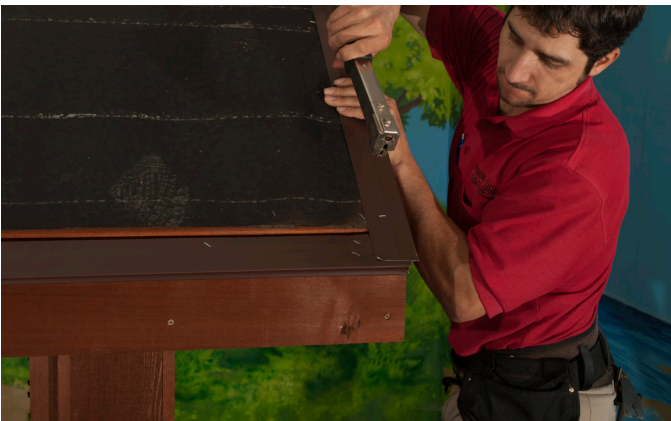
Install Drip Edge on edges using previous steps.
