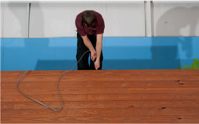
Run Wire through hole drilled in the center of the Ridge.
