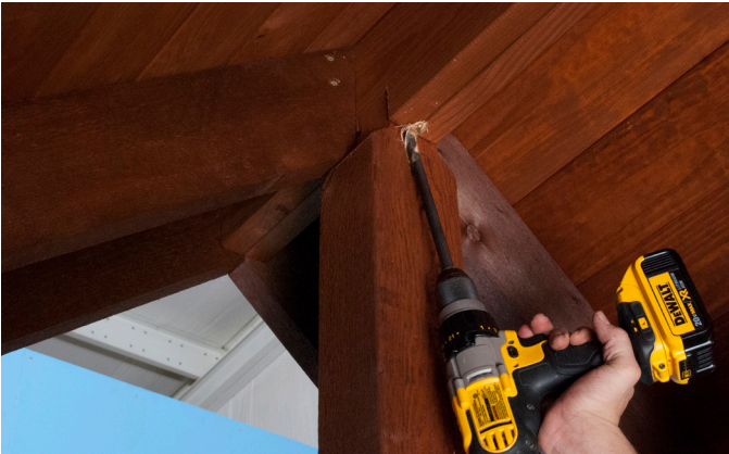
Drill a hole through the Ridge Beam as shown.
