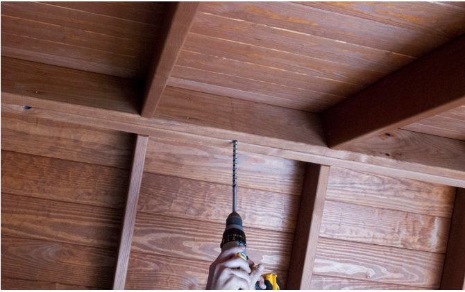
Drill a second hole in the center of the Ridge Beam or desired location.
