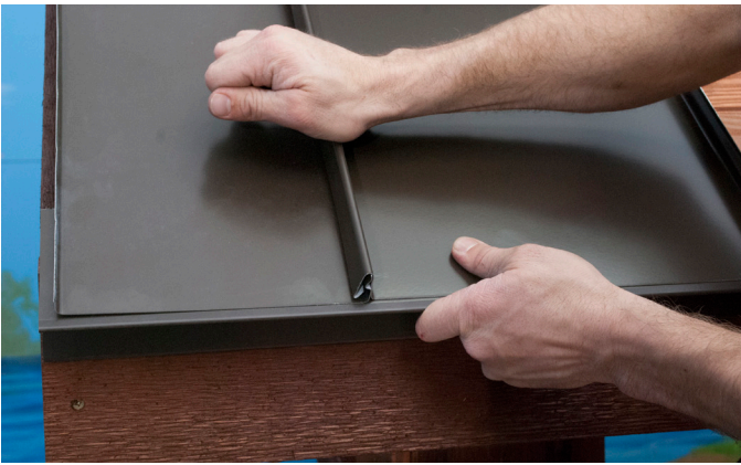
Press down firmly or use a Rubber Mallet to connect the (2) Pieces.
