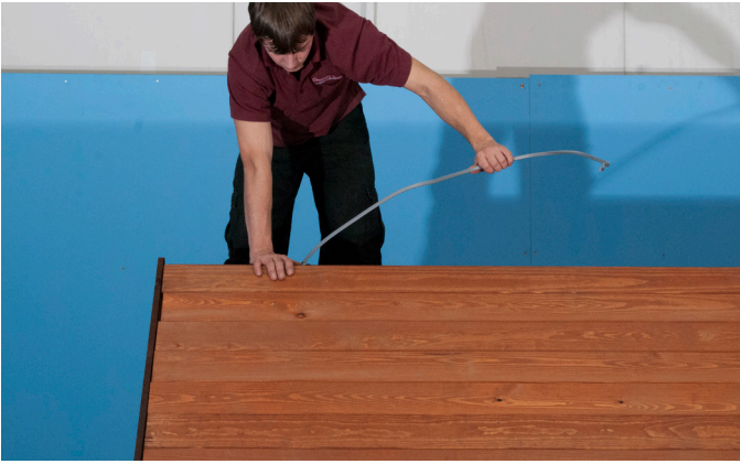
Pull Wire through hole in Ridge Beam.
