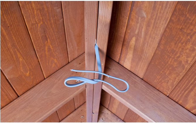
Run Wire out the bottom of Ridge as shown.
