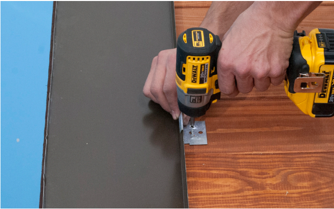
Fasten Metal Clips to T&G using (2) 3/4" Stainless Steel Screws.
