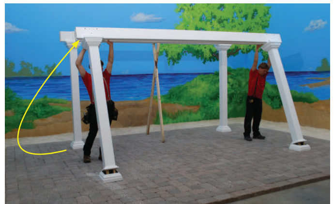
Carefully lay the post side down and lift the header side up into an upright position.
