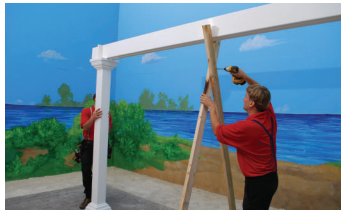
To keep the Header Assembly upright build an A-frame brace using your own 8' long 2x4's and fasten with (2) 2.1/2" screws.
