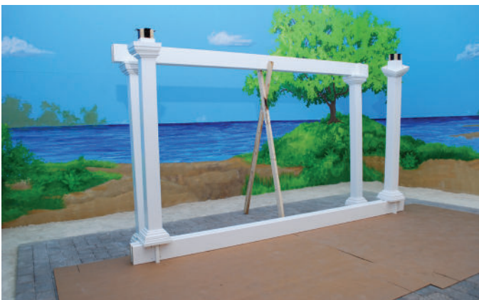
Assemble 2nd Header and Post Assembly in location as shown.
