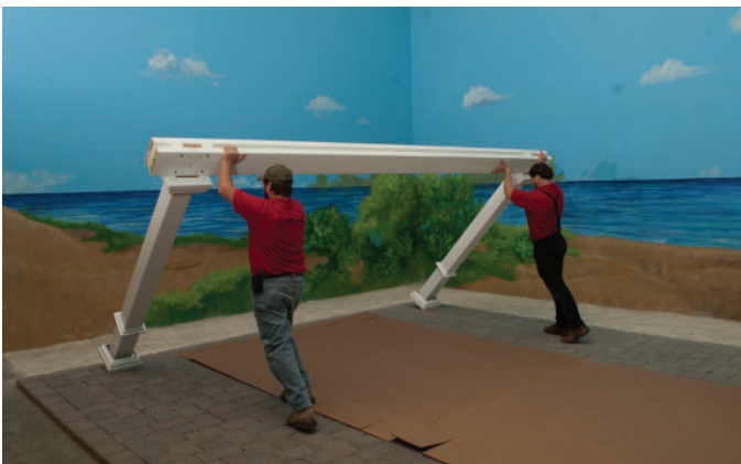
Lift Main Header side up and set into place.
