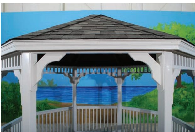
Finish By installing remaining Crown Mouldings.
