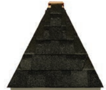
Upper Pagoda Roof Section
