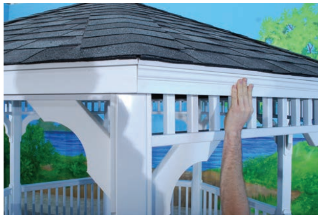
Place Crown Moulding onto Fascia Trim.
