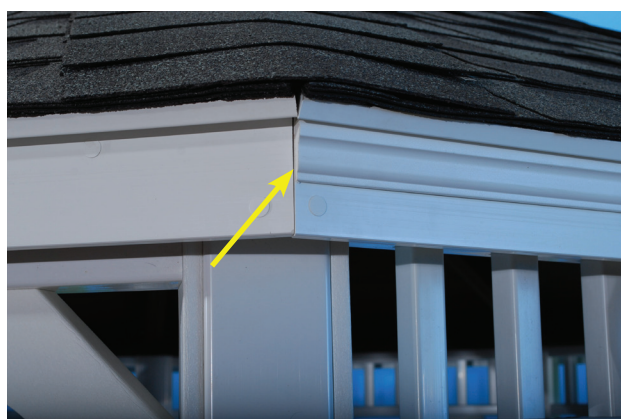
Align Crown Moulding with edge of Roof Panel
