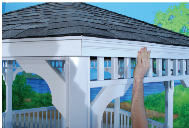
Place Crown Moulding onto Fascia Trim.
