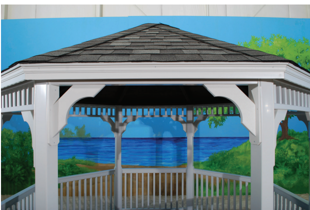
Finish By installing remaining Crown Mouldings.
