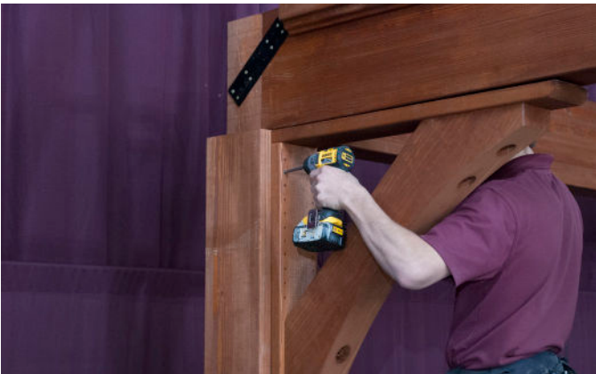
Fasten Brace section to Post and Header using 3 ½" Brown Screws through all pre-drilled holes.
