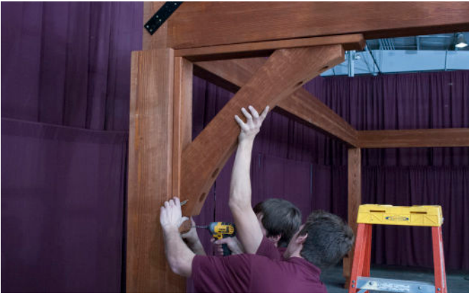
Lift Brace Section into Place.
