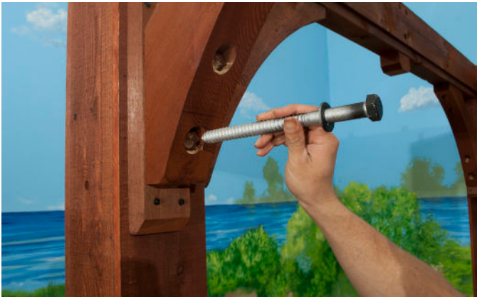
Prepare the 3/4"x10" and 3/4"x12" Lag Bolts with Washers.
