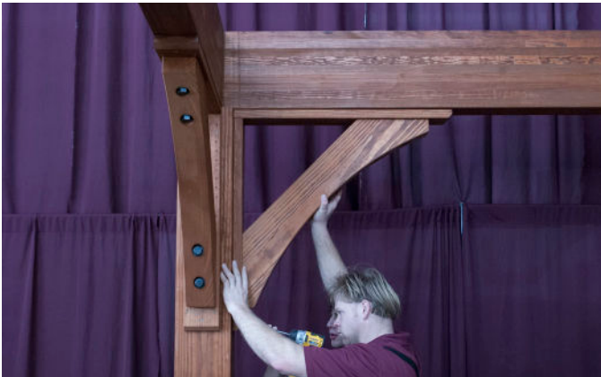
Install all the remaining Brace Sections and Lag Bolts.
