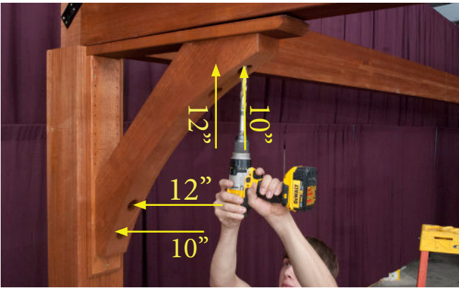
Pre-drill through the Brace and into the Header to the depths shown above for all Posts and Headers. Do not over drill, bit is long enough to come out of opposite side of Post.
