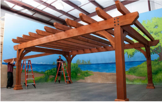
Note the last Rafter is marked.
