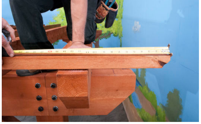
Ensure Stringer is centered on the Rafters with the same overhang on each end.
