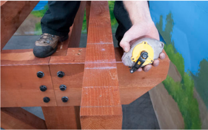
Using a Chalk Line place the line on the pre-marked end rafters.
