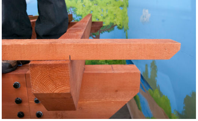
Place the edge of the Stringer flush with marks on the Rafters.
