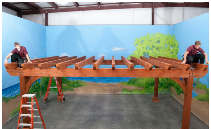
Mark the center Rafters .
