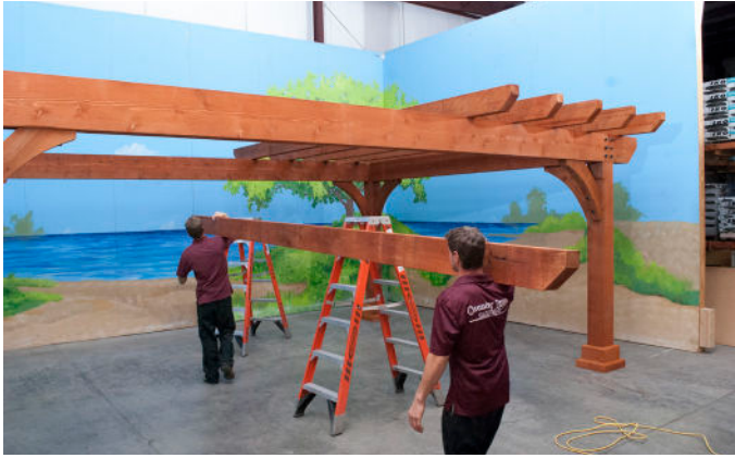
Using Previous steps install remaining Rafters.
