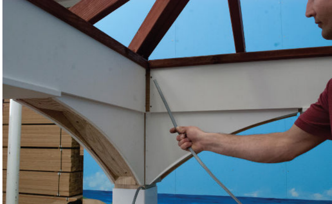
Feed Wire from the post you installed wire in though Top Plate and Double Rafters.
