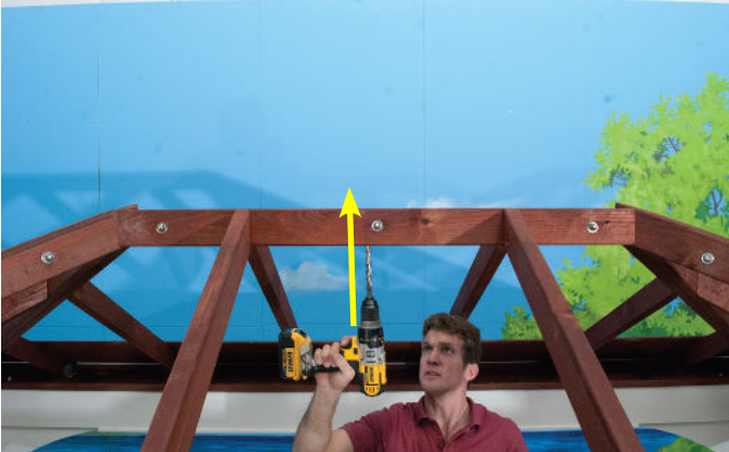
Drill hole through center of Top Ridge.
