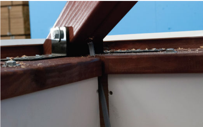
Angle Wire and feed through Corner Rafter.
