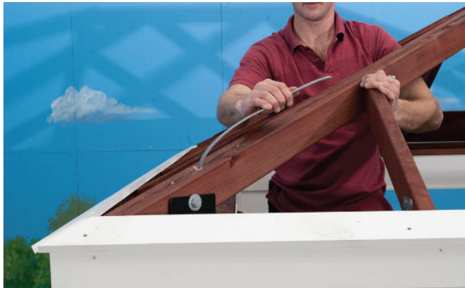
Pull all extra Wire out through hole in Corner Rafter.
