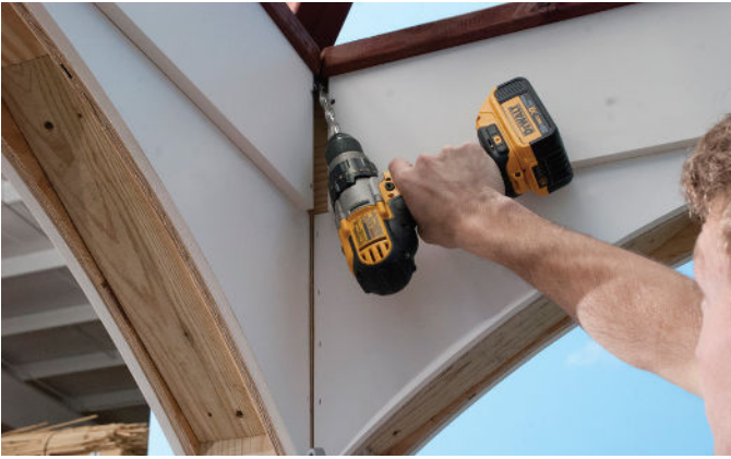
Drill a 1/2" hole through the Top Plate directly below the double Rafter on slight angle towards the corner.
